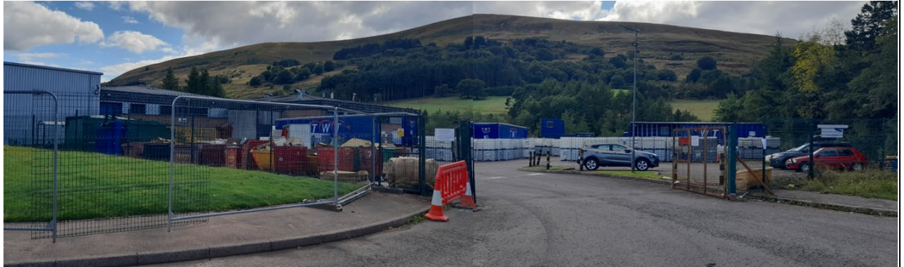
Figure 3- View of the site from the Rising Sun Estate Road.
