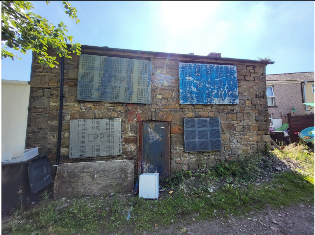
Figure 1.4 Existing front elevation of Calebs Cottage
